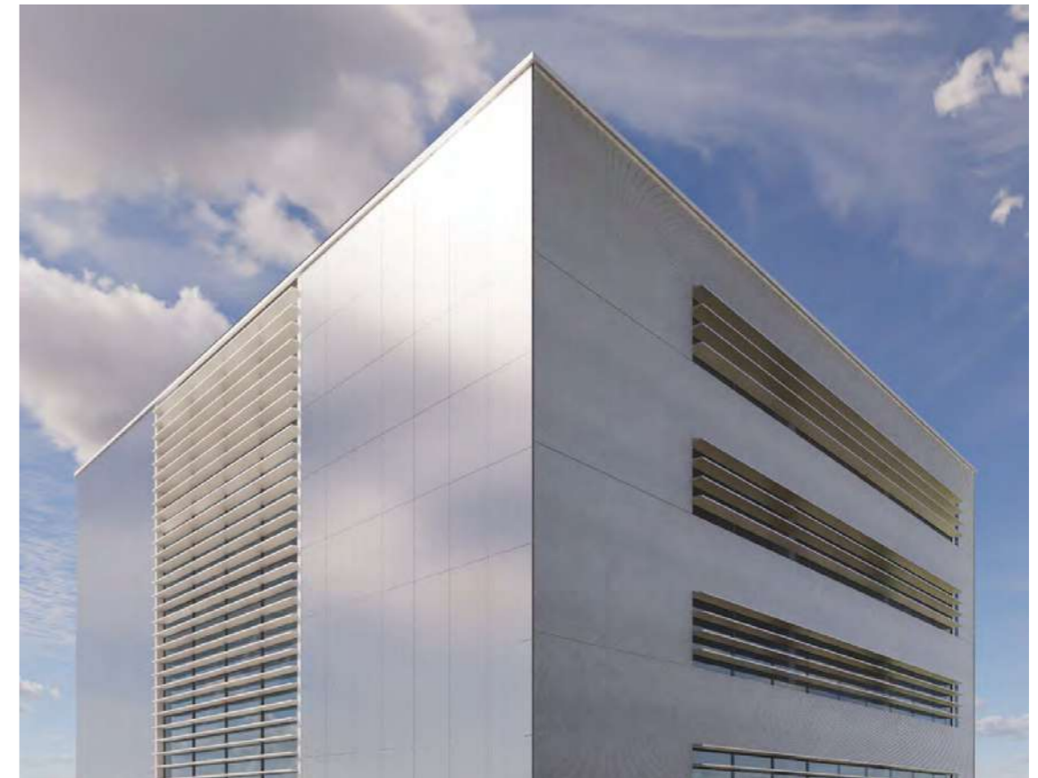
Corner detail with a profile, where new PV South facade meets the old fins design.
